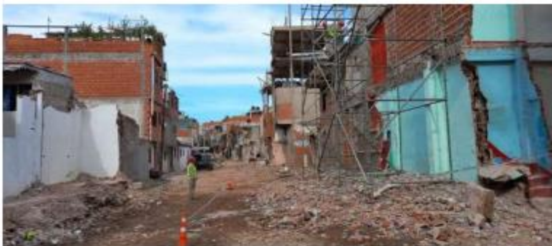
Image 6: Road opening works March 2022 (own picture)
